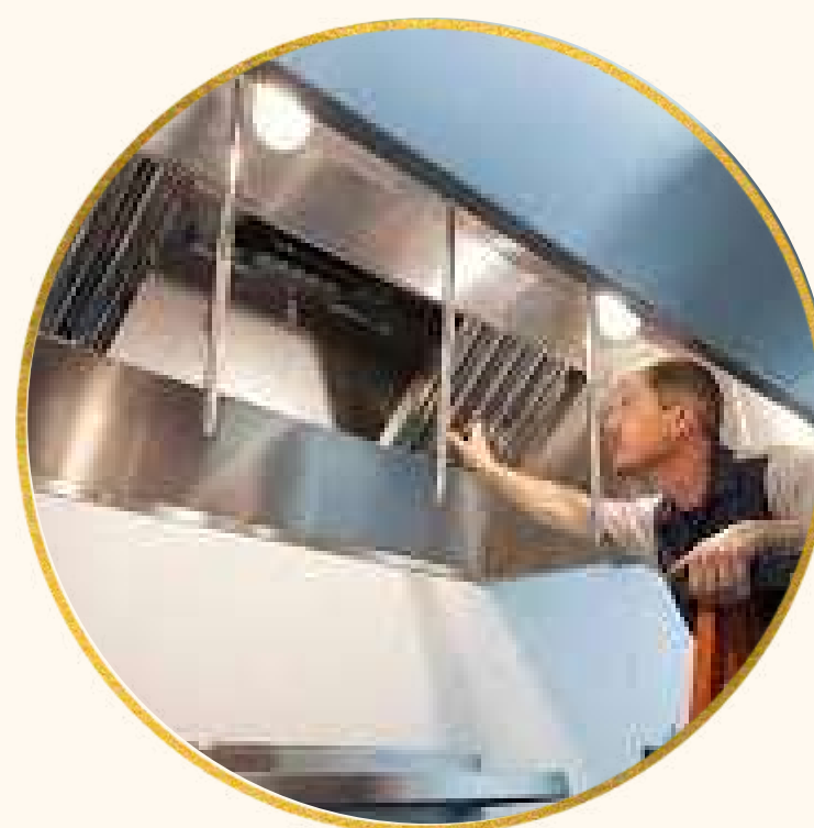
Kitchen Duct cleaning
